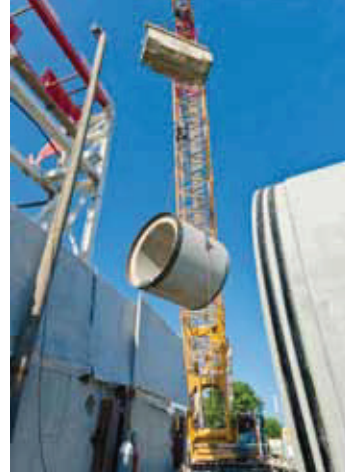
Pipe-jacking construction site using large pipes made of reinforced concrete
